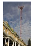
FIGURE 6-22 A WiMAX tower broadcasts signals over a wide area. Subscriber close to the tower can use non-line-of-sight modems to pick up the signal.
